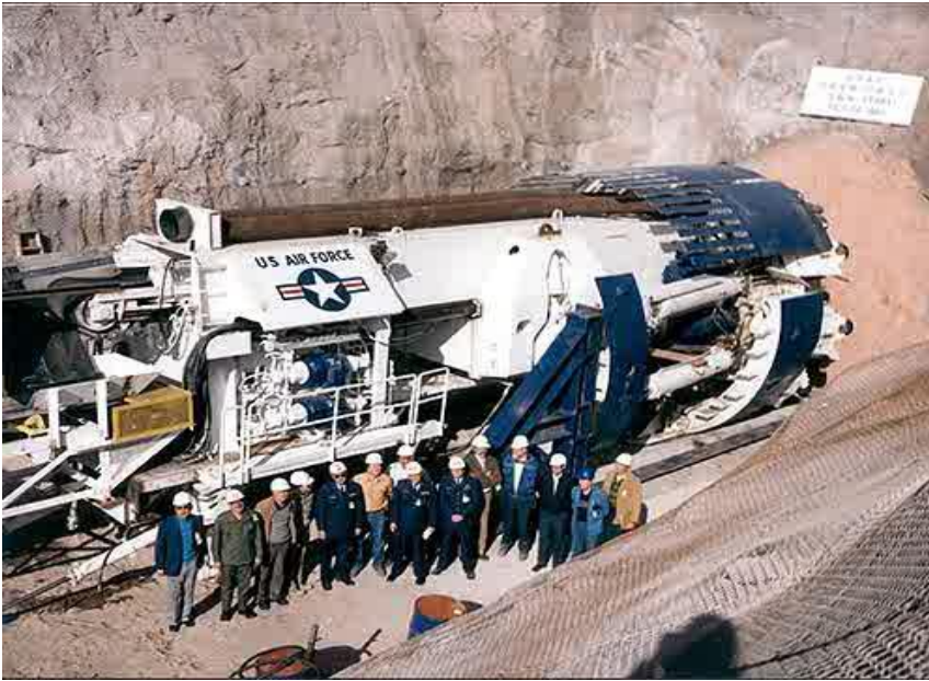
Figure 1. U.S. Air Force tunneling machine, 1982, Nevada. The Air Force has been digging these tunnels for more than 40 years. According to some sources, the newer tunneling machines can dig underground, through 7 miles in one day. Dr Bill Deagle, MD has been quoted as stating that the underground bases are, at least, \frac{1}{4} of a mile underground. The author's personal experience concludes that the tunneling program has been extended to other cities in the United States.
